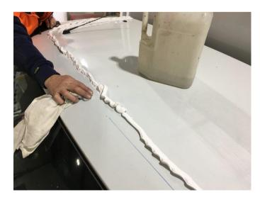
3. Lightly abrade the cab surface using 240 grit sandpaper 10mm inside the outline of the kit. Apply a heavy line of Urethane glue to the cab roof in the areas shown, then clean the texta lines off.
