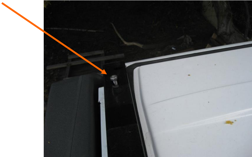
Rear Roof Support Frame
